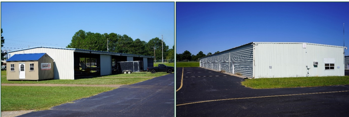
T-Hangar Facilities at TXK
