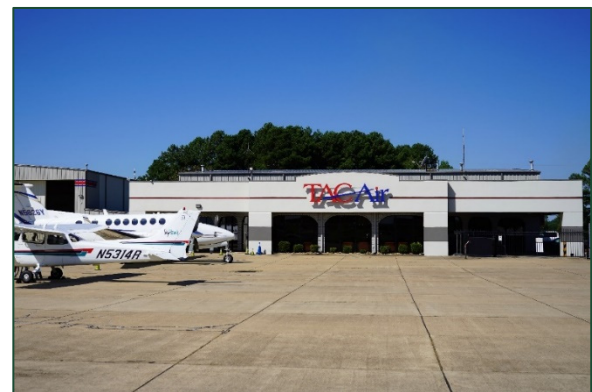
FBO Terminal and Ramp (Note: Signature Flight Support now owns this facility)
