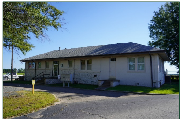
Airport Administration Building
